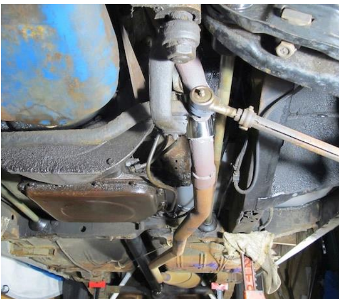
It's easy to see how badly the exhaust shop bent the smallish/restrictive exhaust.
